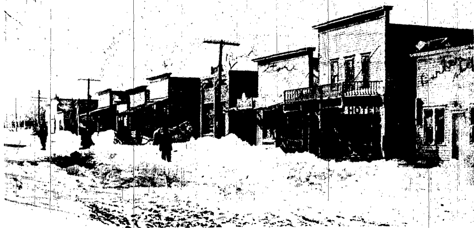
EARLYDAY HOSKINS appeared like this following a storm. The year was not given. Mrs. Erwin Ulrich supplied the picture. Identification of some of the places had been penciled in on
